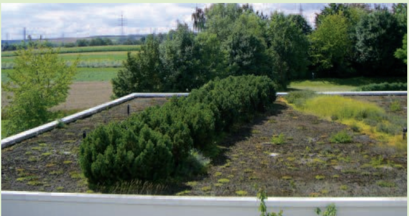
An intensive green roof
