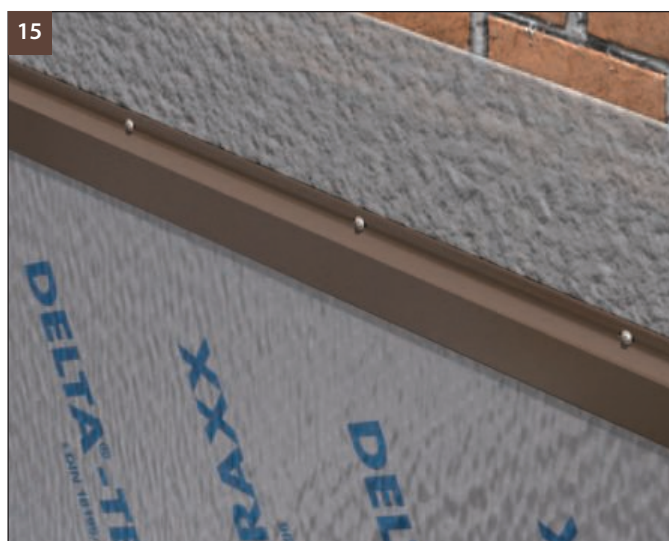
(Fig. 15) Protect the sheet with DELTA ® -NOPPENBAHNEN-PROFIL and cover the fastening points.
