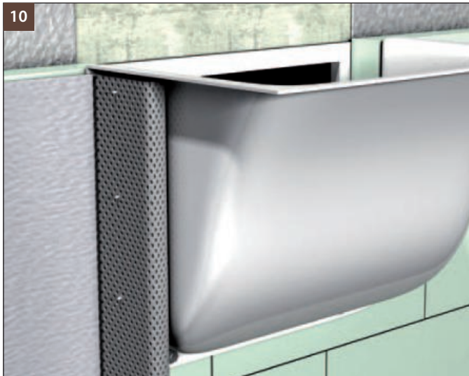
(Fig. 10) When light wells have already been installed, cut the sheet precisely along the lower edge, make one vertical cut in the middle, and attach the projecting ends with adhesive pins.
